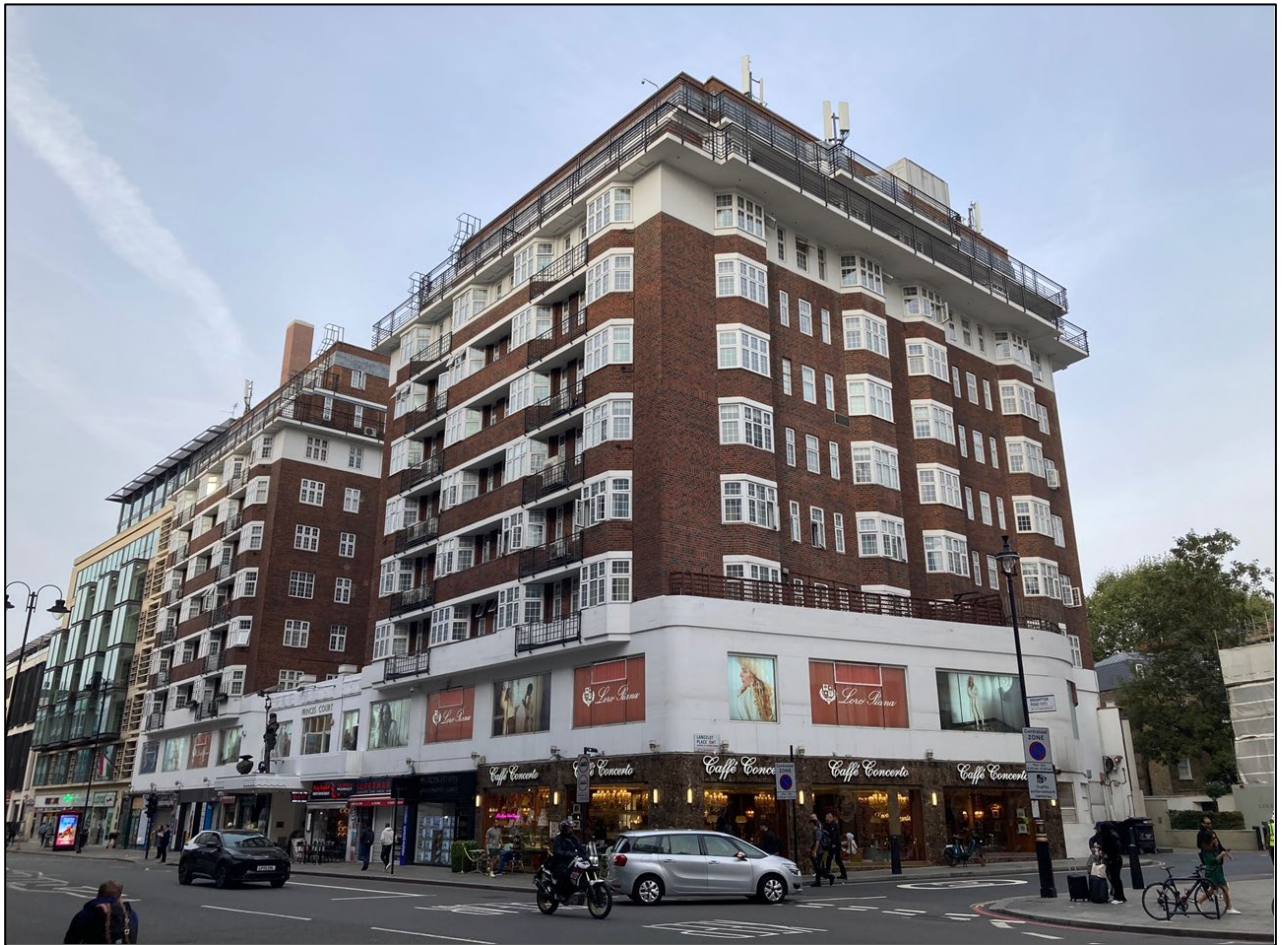
Exterior of Princes Court. Application site is first floor level.
