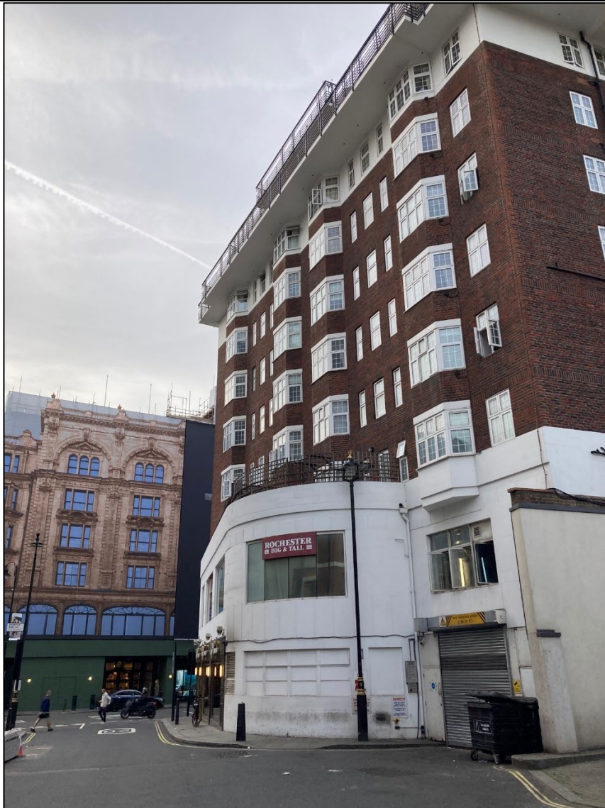
Exterior showing entrance to shared service yard and relationship of application site with Harrods.
