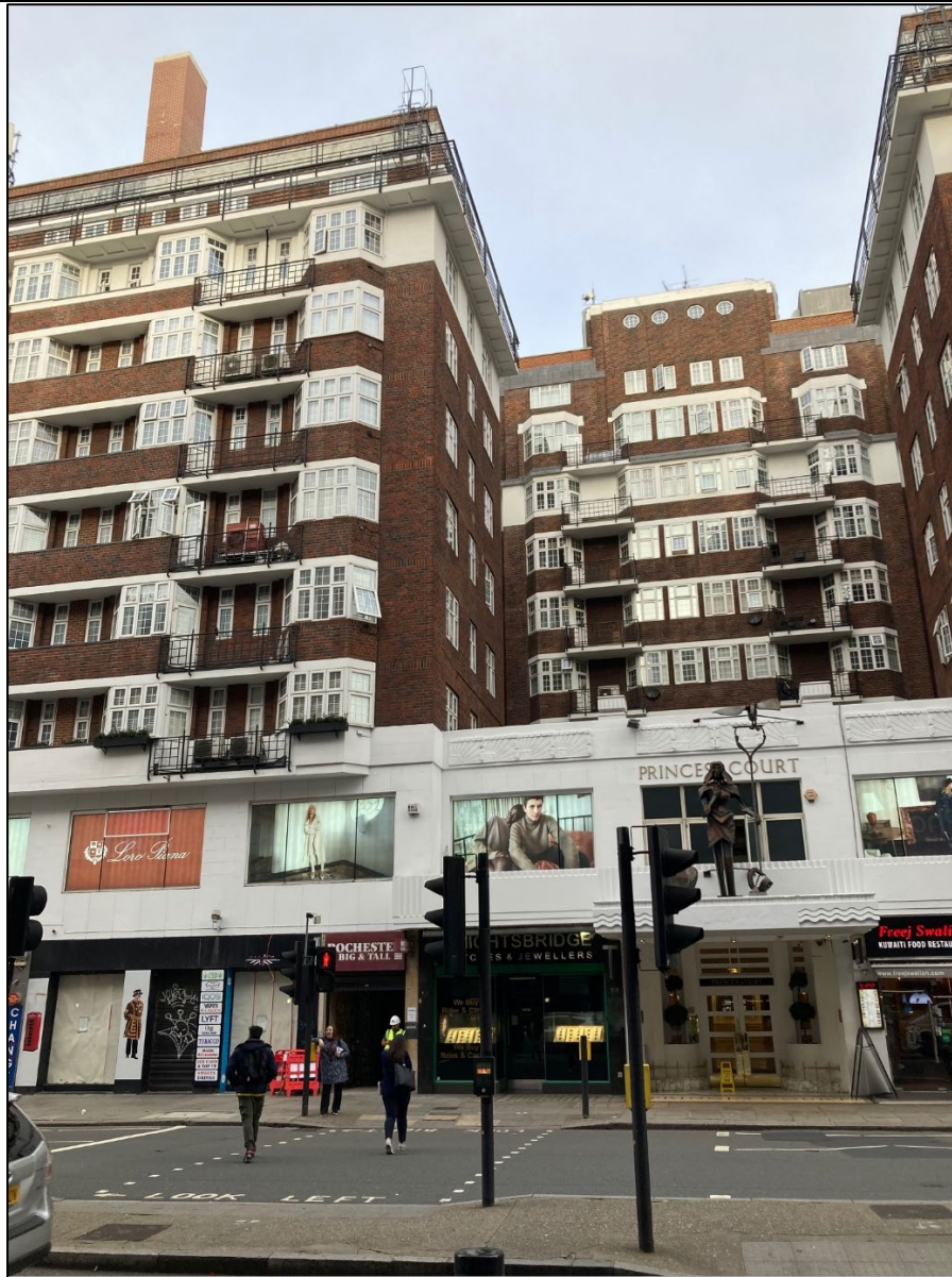
Exterior showing ground floor entrance to subject site (beneath “Rochester Big & Tall” sign).
